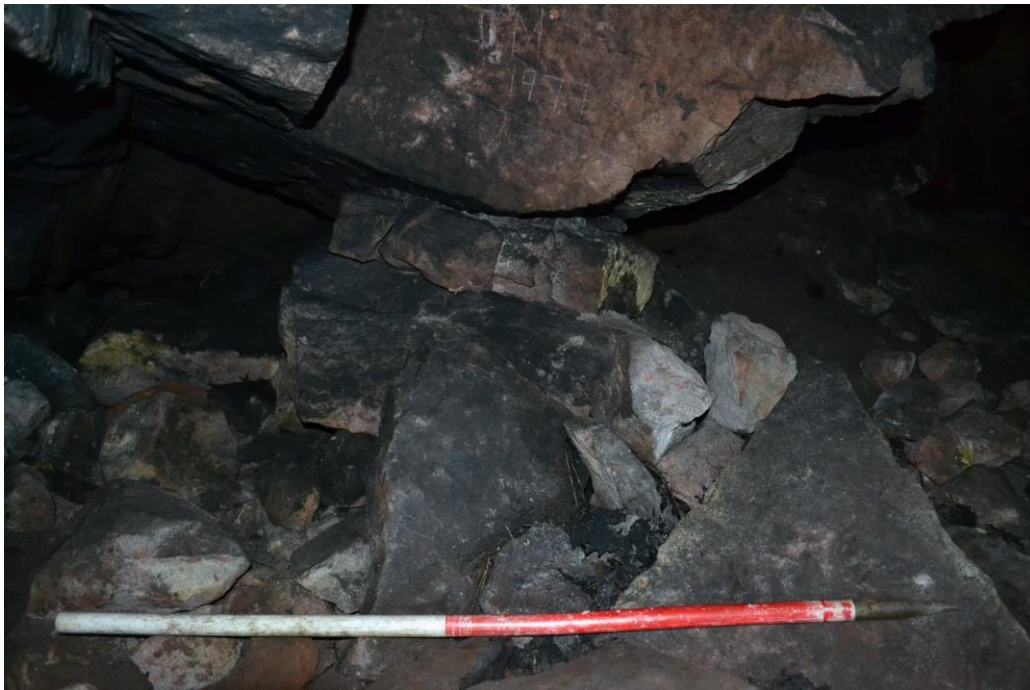
Illus 15: The drystone masonry pier on the east side of the main chamber of Well Cave.
