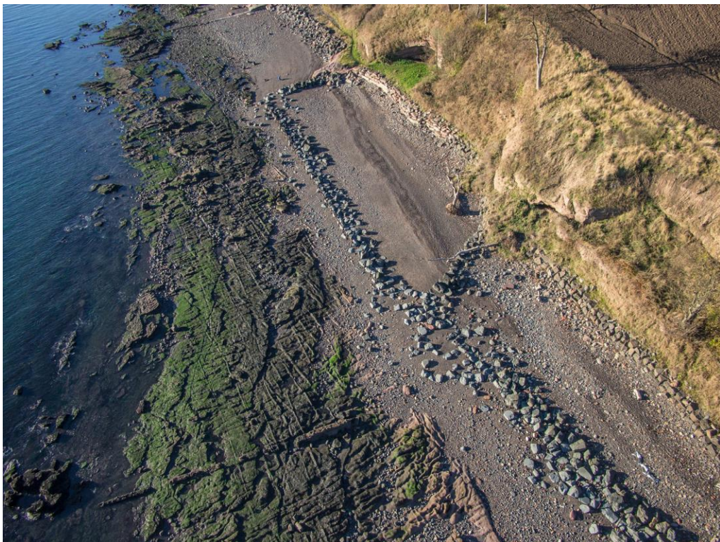
Illus 36: Sea defences (Interventions 6 and 7, Table 5) and dispersed rock armour with surviving iron elements of groynes (Intervention 14) in front of Jonathan's Cave (Eddie Martin 2013).
